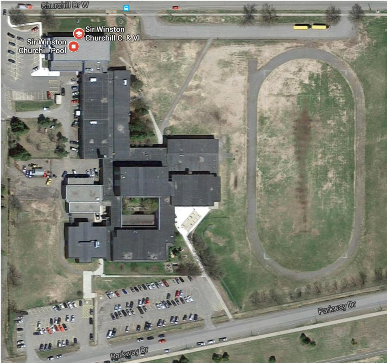
Aerial View – School Site
